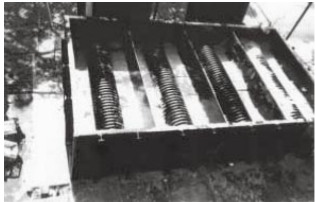
Figure 2. Soil chambers (half full) after compaction
