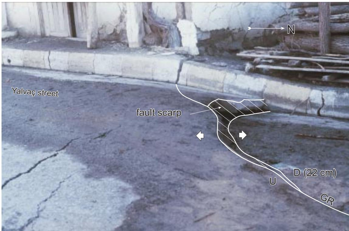
Figure 15. General view of the Çay ground rupture that cut the NNW-trending asphaltic Yalvaç street and down-dropped it as much as 22 cm (view towards west). U– up-thrown block and D– down-dropped block (hanging-wall block).
