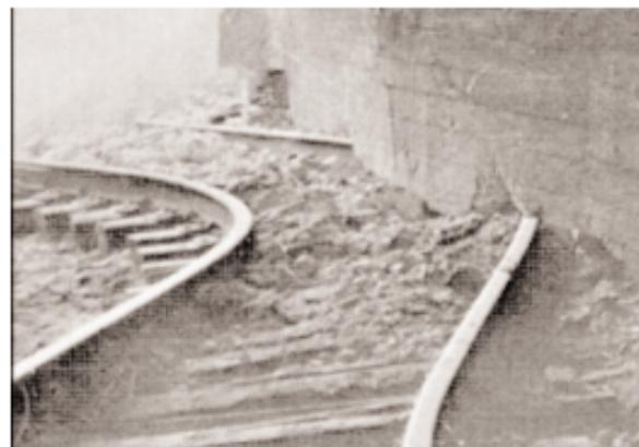
Figure 3. Bent rails inside the Kern County urban railway tunnel. The White Wolf Fault had a both compressive and lateral dislocation during the 1952 Kern County earthquake. Indicative of this type of fault dislocation is the fact that the rails are bent and continuous underneath the tunnel wall, showing that the wall was lifted up enough for the rail to slide underneath. Source: SCECDC 2002.
