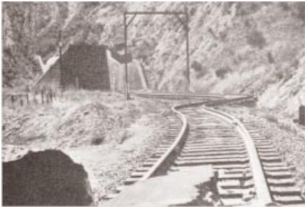
Figure 2. Kern County urban railway tunnel. A view from the entrance of the tunnel showing bent rails near a zone of intense fracturing along the White Wolf Fault. Source: SCECDC 2002.
