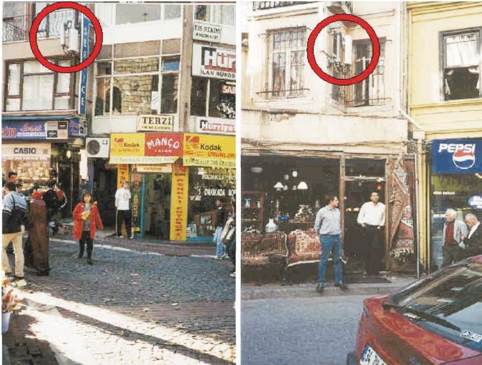
**Figure 1.** Two base station antenna locations in Kadıköy (in Istanbul). Measured electric field strength on the ground varies between 2 V/m and 6 V/m.
