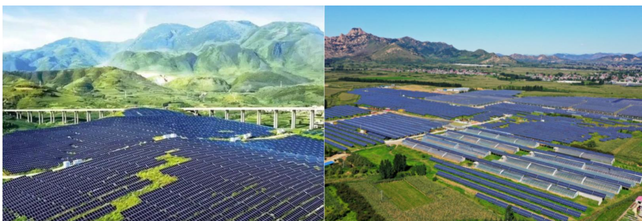
Figure 2. Photovoltaic systems exposed to complex environments in farmland.
