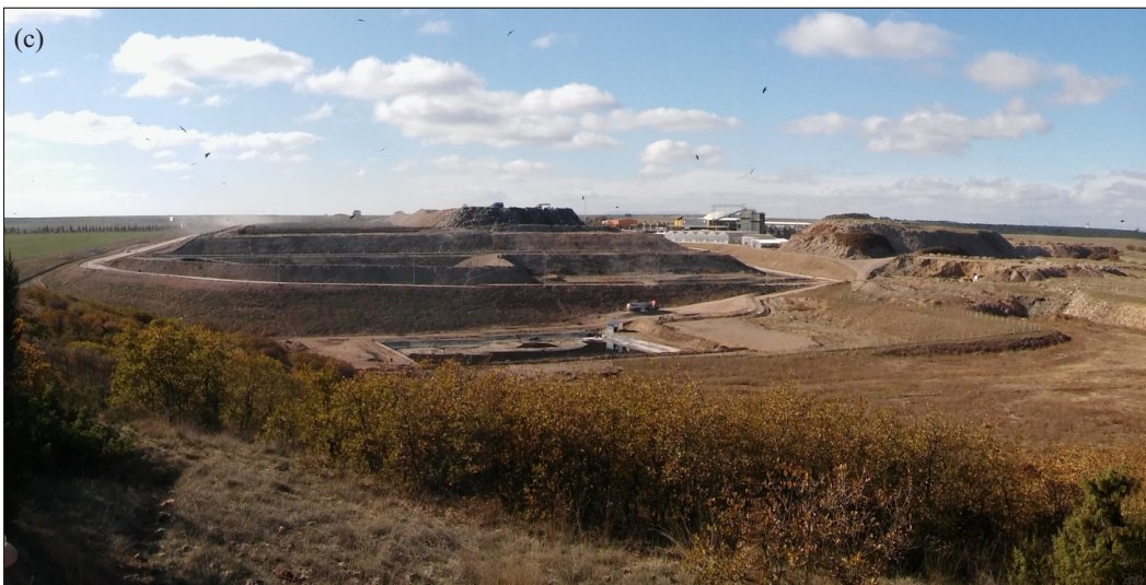
Figure 5. View of the Eskişehir regular landfill from (a) west to east, (b) south to north, and (c) north to south.
