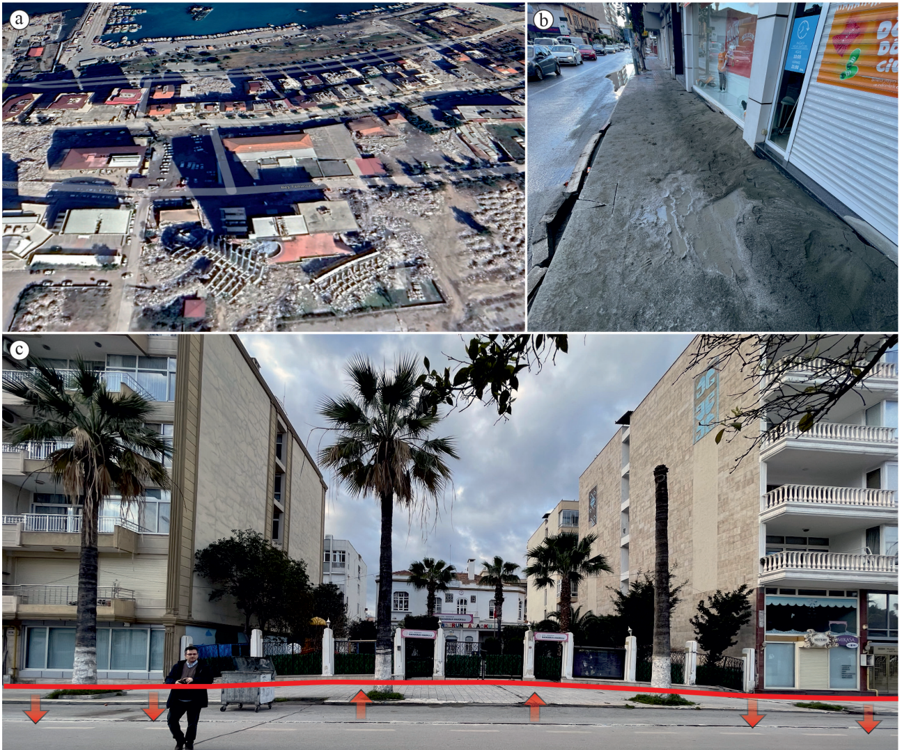
Figure 13. a) Collapsed tall buildings along the İskenderun Bay due to the soil liquefaction, indicating weak soil conditions along the sea shore (Google Earth picture). b) Liquefaction-related sand ejecta from the soil along the buildings. c) Relatively low subsidence area between two subsided tall buildings along the İskenderun coastal zone.
