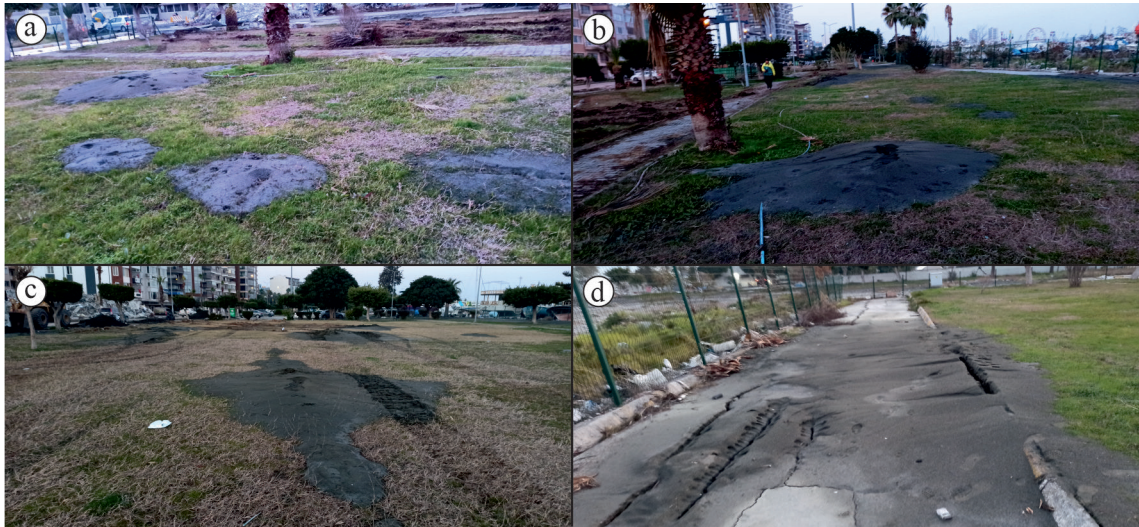
Figure 6. Silty sand cones formed in parks, at the base of poles, and around foundations along the shoreline. These resulted from water-soil slurry ejected from the ground due to liquefaction. Image locations are indicated in Figure 3.
