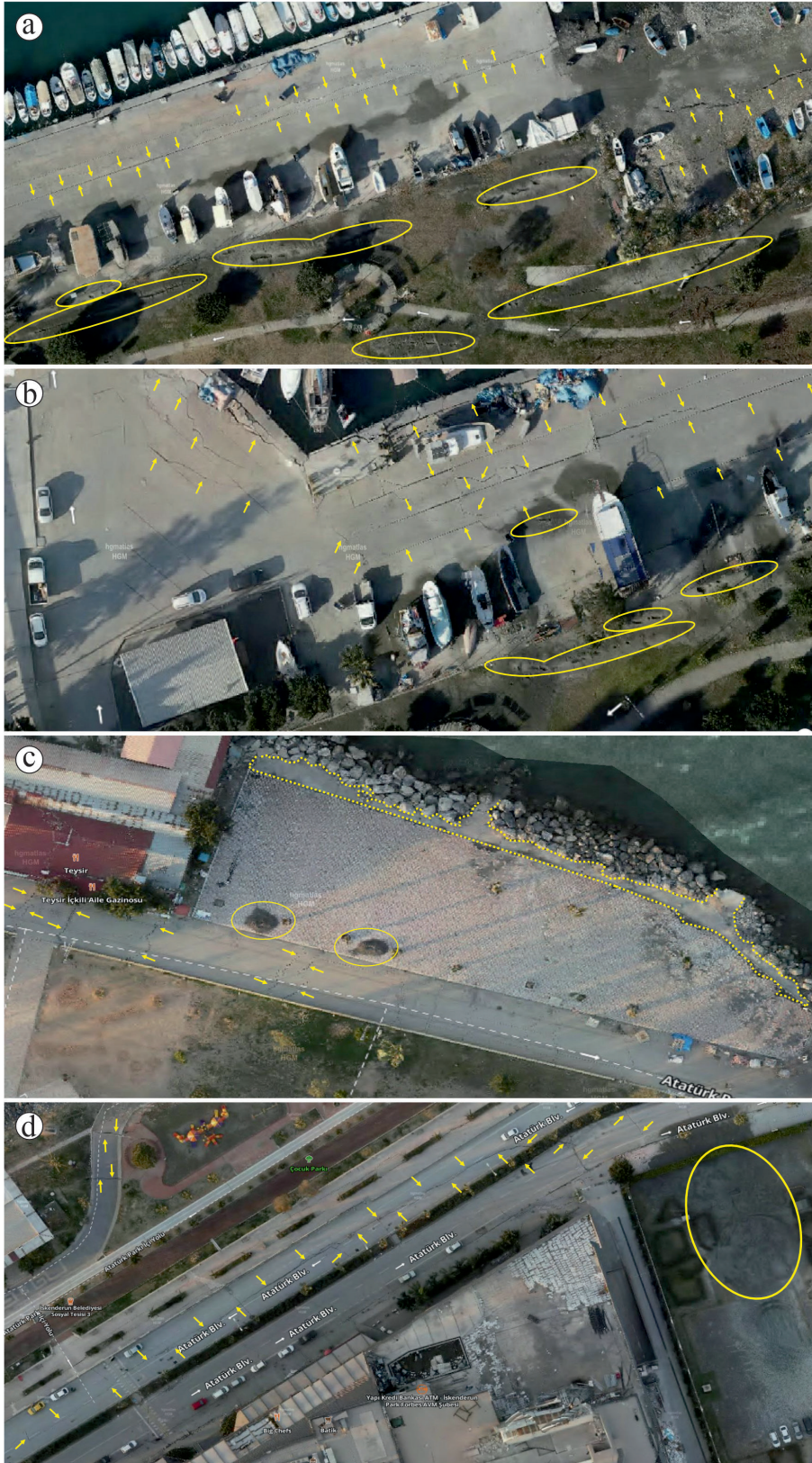
Figure 9. Yellow arrows show lateral spreading cracks and circles indicate sand ejecta associated with the main earthquake.
