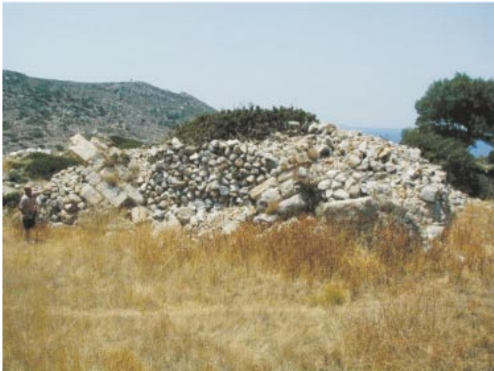
Figure 7. Collapsed building north of the main E–W street.
