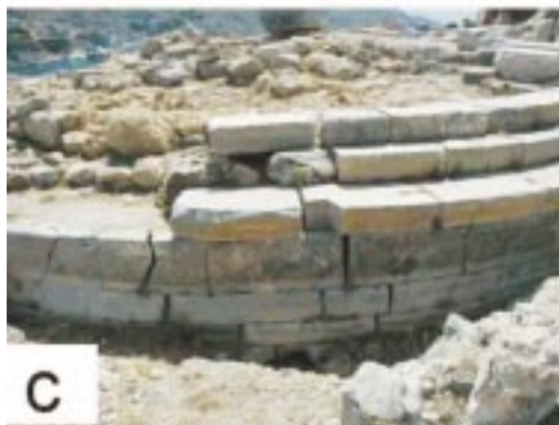
Figure 5. (a) Plan view of the podium of the Round Temple of Aphrodite Euploia showing the trace of a crack that bisects the structure, from Love 1972b, figure 6). (b) Close-up view of the southwest side of the podium showing vertical offset and dilated blocks that accommodate a net 0.5-m downthrow of the southern side. (c) Close-up view of the northeast side of the podium. (d) View to the northeast showing the bedrock fault that juxtaposes limestones with alluvial terrace materials and cuts directly through the podium.
