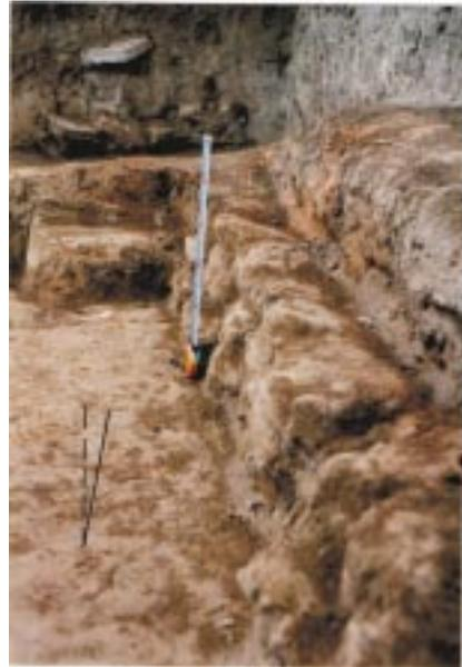
Figure 8. Shift and tilt in a northeast direction of lower course of masonry of *saman* bricks in room No. 16. Angle of declination of deformed wall is between the solid line (modern wall inclination) and the dashed line (originally vertical wall).
