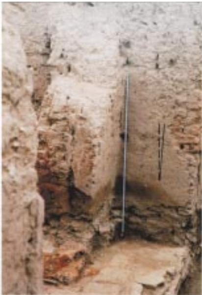
Figure 12. A SW-tilting column support of the entrance into the central chamber of the Buddhist temple.
