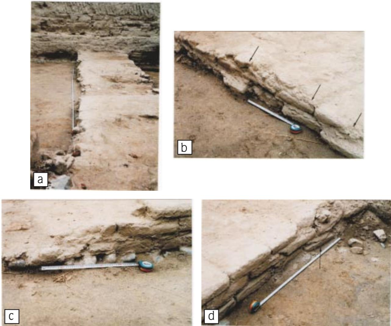
Figure 14. Deformation of the "podium" in the central room of the Buddhist temple: (a) uneven edges of the podium; (b) shifting of individual bricks; (c) "seismic buffer" of the podium, consisting of pebbles and reeds; (d) the shift and clockwise rotation of one of the bricks of the podium.
