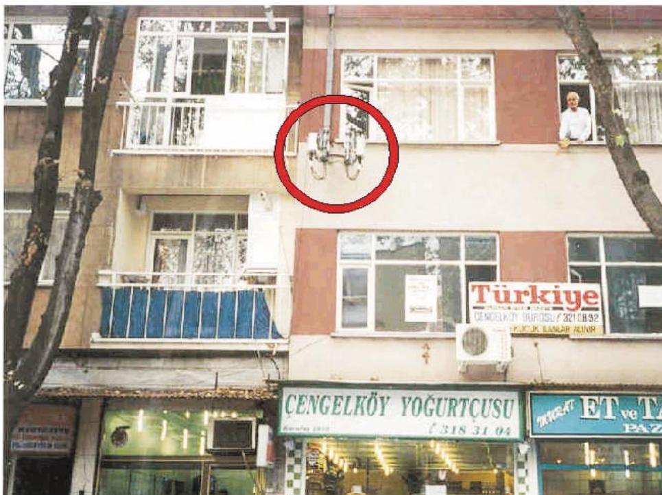
Figure 2. Another base station antenna in Cengelköy (in Istanbul). Measured electric field strength on the ground varies between 3 V/m and 13 V/m.
